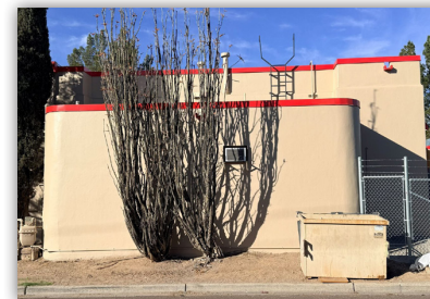
Fire Station 2 east-facing wall
