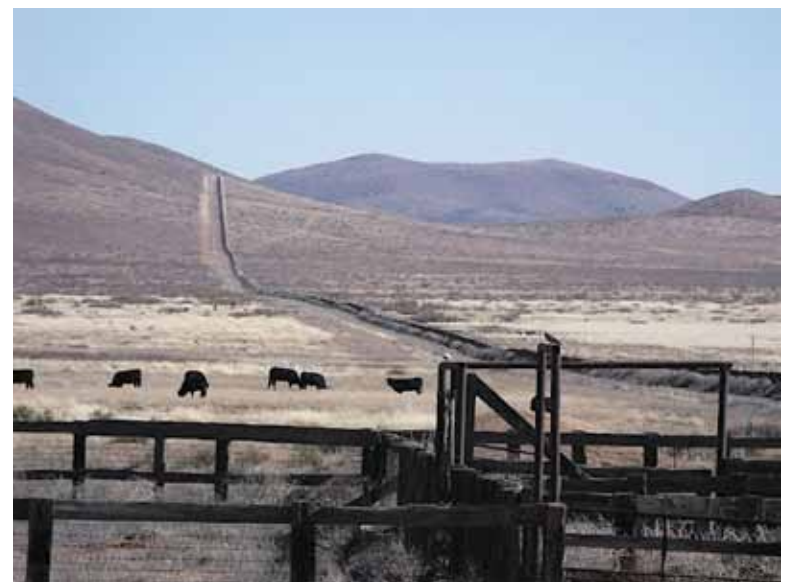
New vehicle barrier extending toward Columbus and the "historic" corral at Antelope Wells, constructed when President Ulysses S. Grant opened the port of entry, according to the local legend.
