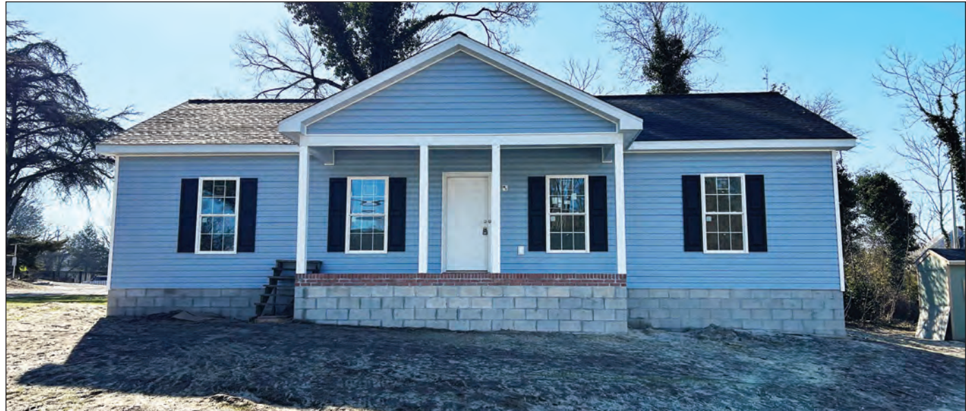
A Habitat for Humanity of Wicomico County house under construction. PROVIDED
