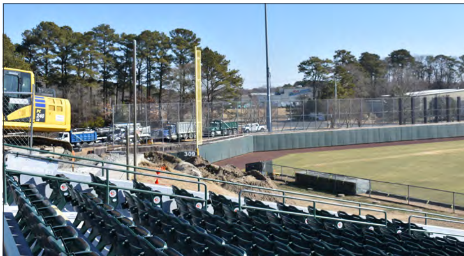
Construction is underway on a new 9,000-square-foot indoor performance center.
