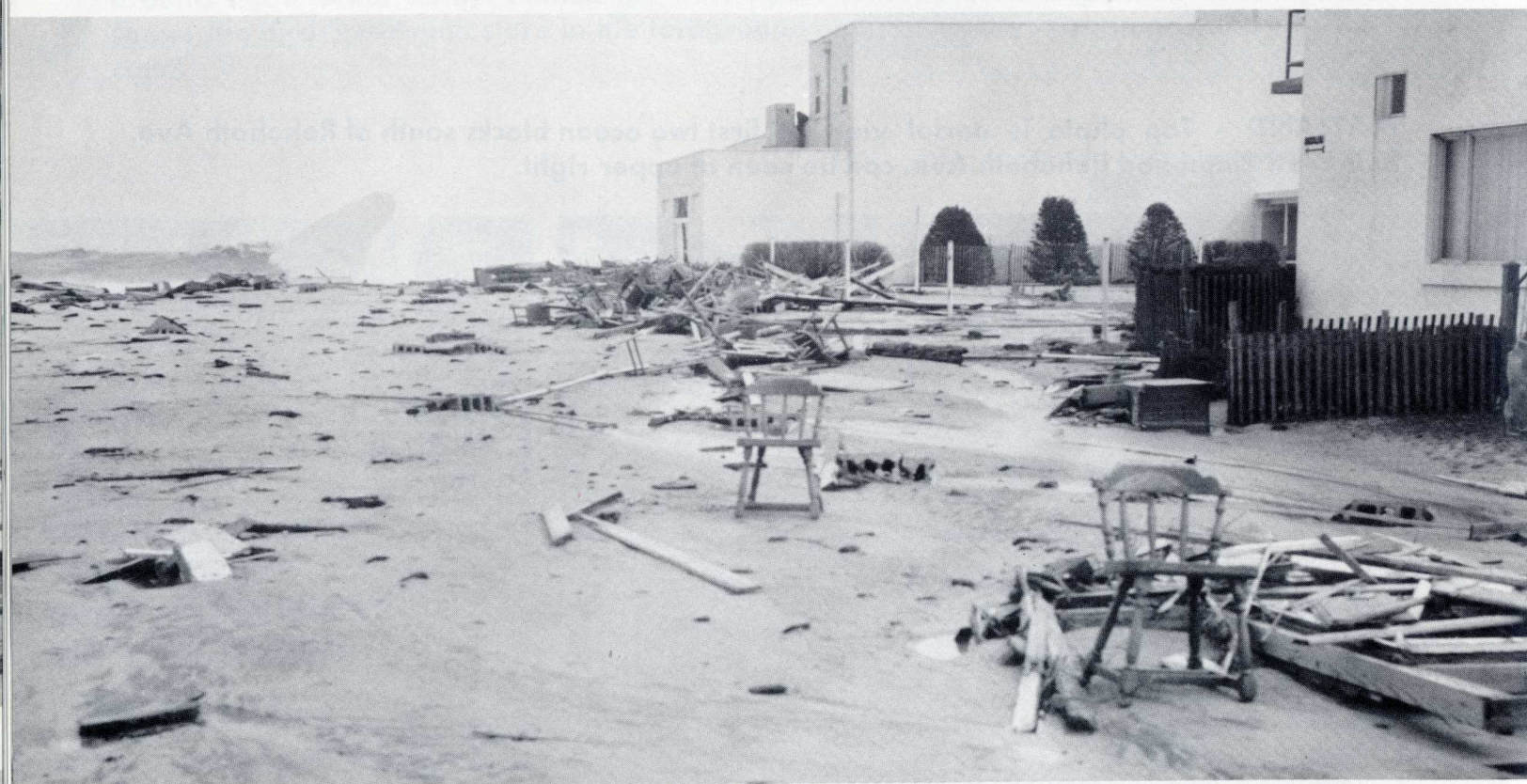
GRIER HOME - Just north of the Henlopen Hotel the ocean cut out Surf Avenue and undermined the Grier home. House on corner has fallen into the sea. Bottom, photo taken from the side of the Henlopen Hotel looking east. Notice cinder blocks and furniture washed back by the sea.
