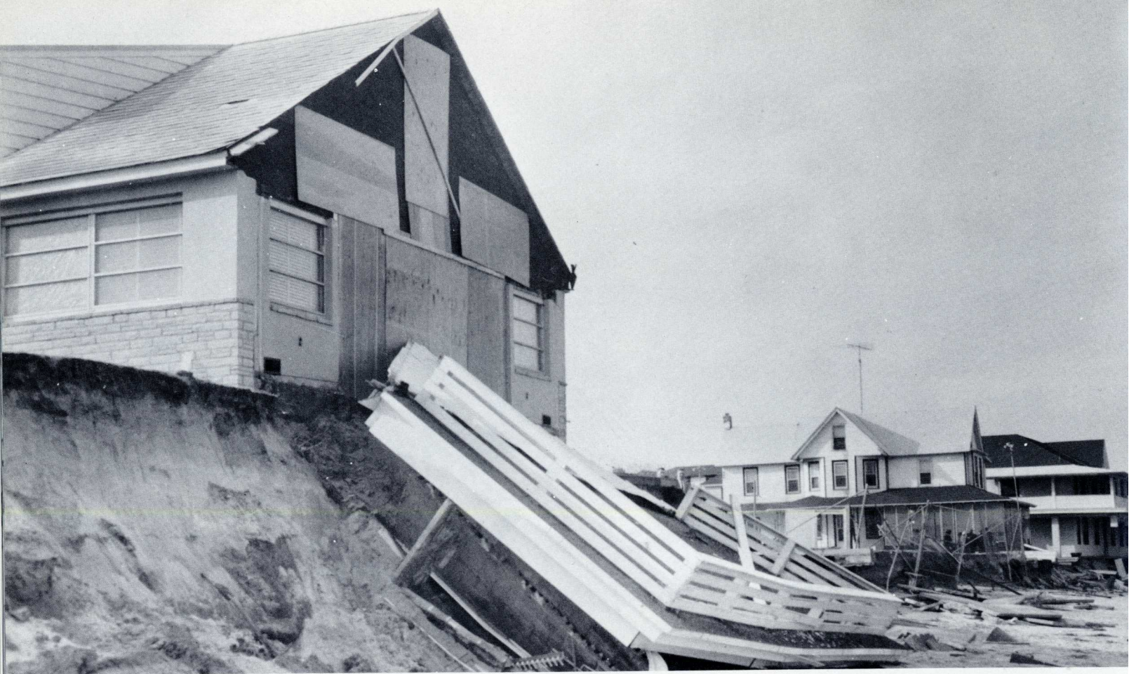
REHOBOTH - Top photo shows the Raymond Goslee home at the foot of Philadelphia Avenue and Boardwalk. Bottom, unidentified, shows force with which seas twisted wall sections and broke out block foundations.
