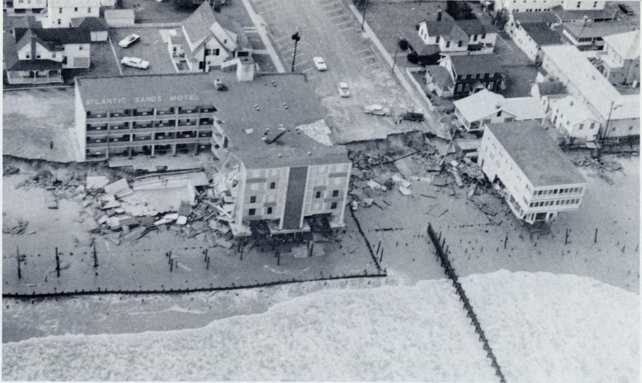
MARYLAND AVE. & OCEAN - The Atlantic Sands Motel shown in this aerial view suffered extensive damage. Notice swimming pool undermined in lower left corner. Entire front wing of motel was undermined and additional sections fell after this picture was made.
