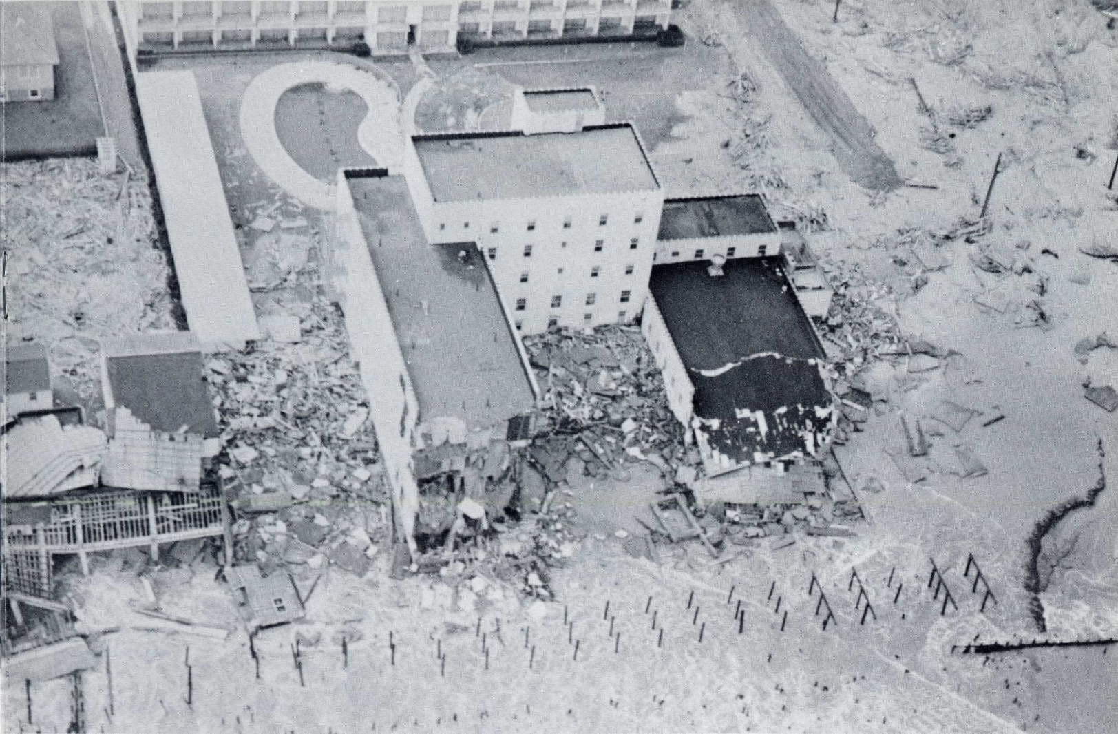
HENLOPEN HOTEL - This aerial view shows the extensive damage to Rehoboth's largest hotel on the right and the Stuart-Kingston Gallery on the left. Lower picture is view of Surf Apartments at the foot of Olive Avenue.
