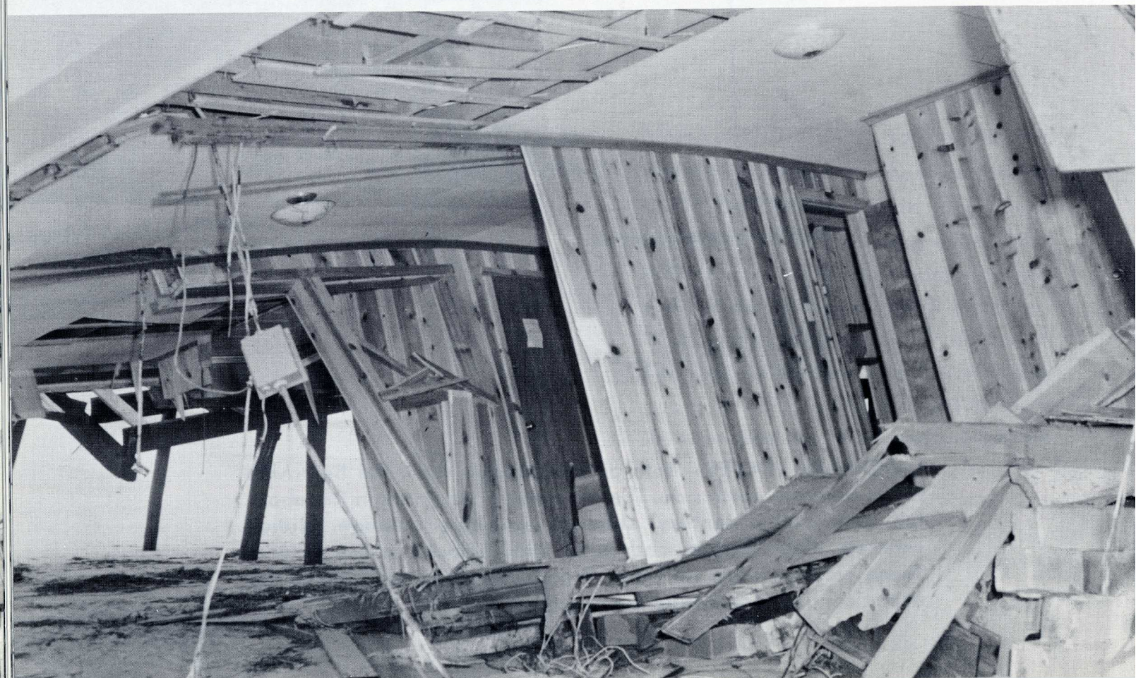
REHOBOTH - Top photo shows the Raymond Goslee home at the foot of Philadelphia Avenue and Boardwalk. Bottom, unidentified, shows force with which seas twisted wall sections and broke out block foundations.
