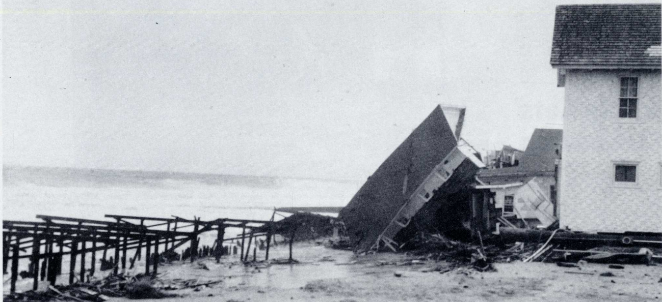
GOING - GONE- Top photo was taken north of Dolle's looking south. Bottom photo taken from the same location a few minutes later shows the apartments over the Dolle's store fall to the beach.
