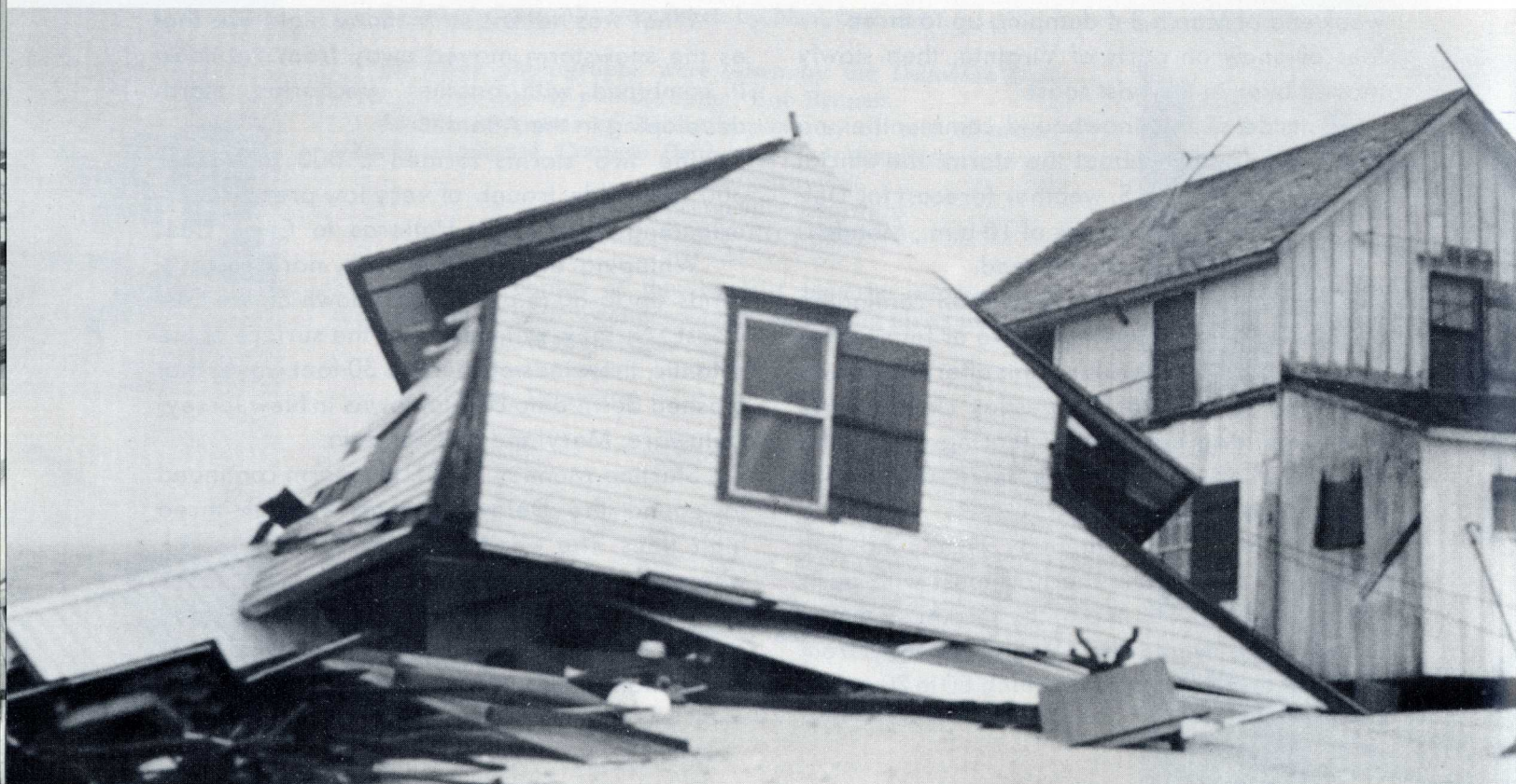
BOWER'S BEACH Tuesday afternoon - a bay-front house collapsed and street scene littered with debris. Many homes along the Delaware Bay front were floated free of their foundations and pushed by the tides and wind a mile or more onto the marsh.
