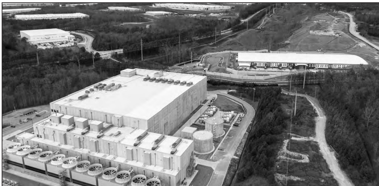
Pictured is an aerial photo of new expansion of Douglas County's Google Data Center (foreground) and a construction site of the new data center Switch (background) in Lithia Springs, Georgia, on Jan. 17, 2020.
