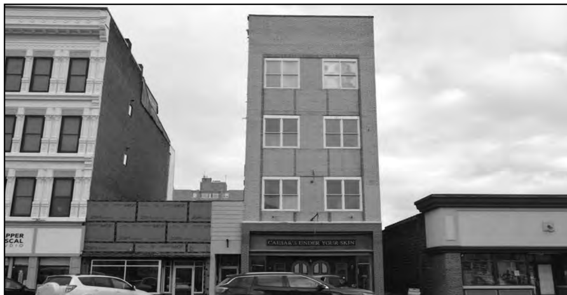
The city's Downtown Revitalization Initiative calls for beautifying the city with art and redone building facades. Cortland Mayor Scott Steve said this facade, at 89 Main St., is up for renovation this year.
