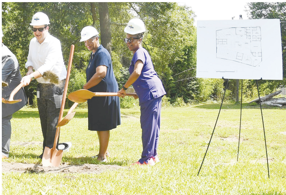
Members in the Community: Library ground-breaking
