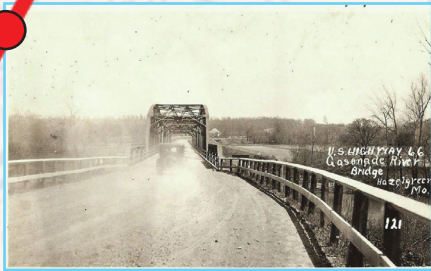
MILE 2.1 - THE GASCONADE BRIDGE
