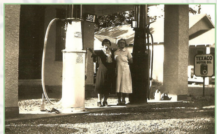
MILE 31.0 - TWIN OAKS STATION
