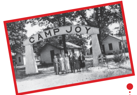
The arch at the entrance to Camp Joy, one of Lebanon's first tourist camps.
