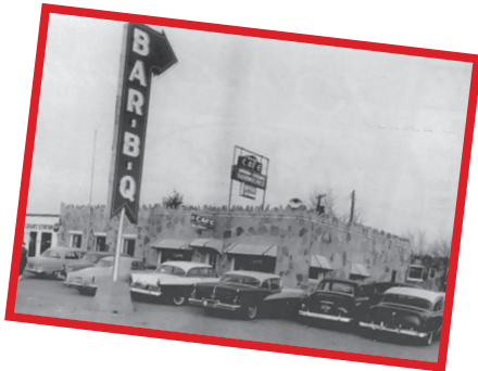
The Rock Court, which included a barbecue restaurant, was located on the south side of Route 66 just west of the Munger Moss.
