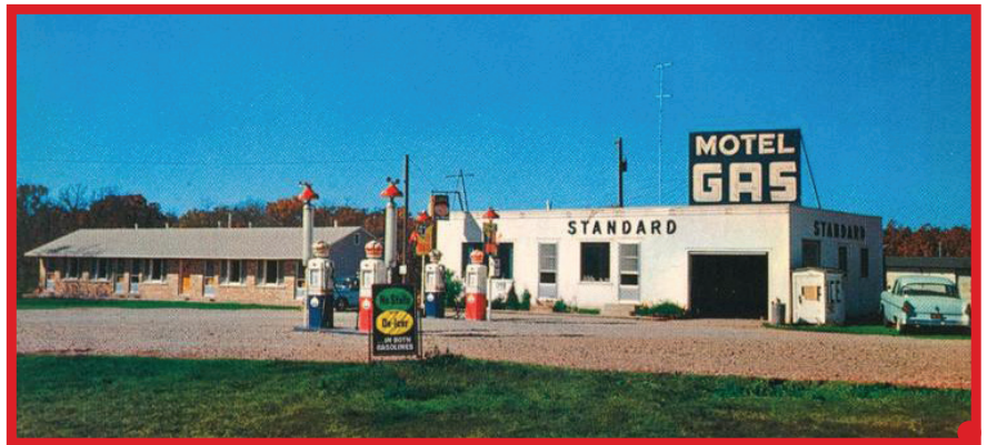
The Midway Motel and Standard Station on Route 66 at Phillipsburg, pictured in the late 1950's after the opening of New Route 66 and Interstate 44. The back of the postcard advertises these features: "Tiled Bath — Air Conditioned — Panel Ray Heat — Cafe — Gifts — Standard Gas — Reasonable Rates — Quiet — off The Highway." Originally, this was the site of Midway Cafe and Camp. The Standard Station, later remodeled for other business uses, was destroyed by a fire several years ago. The motel, converted to storage units, was torn down in 2017.
