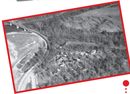
Aerial view of the Gasconade River Bridge pre-interstate 44.
