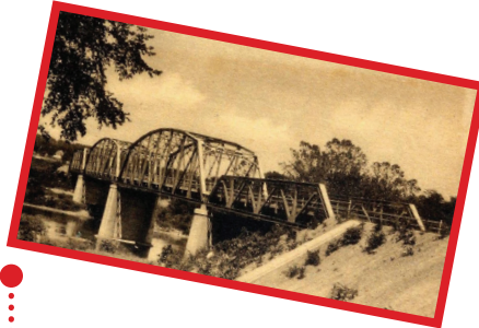
Route 66 Gasconade River Bridge at Hazelgreen.
